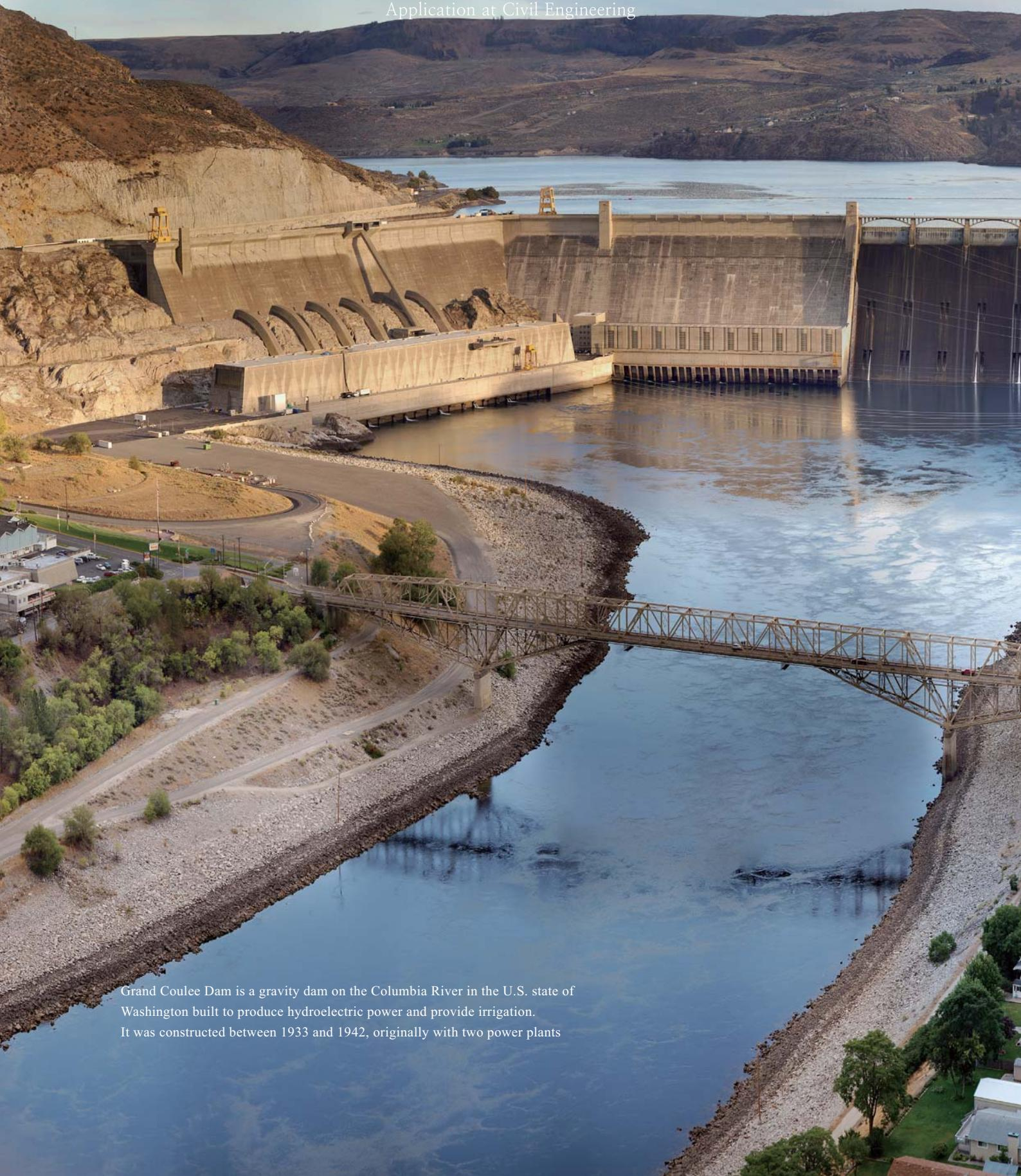
Grand Coulee Dam is a gravity dam on the Columbia River in the U.S. state of Washington built to produce hydroelectric power and provide irrigation.
